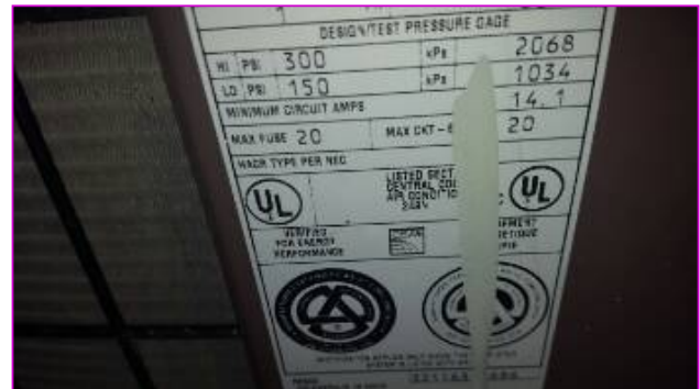
Unit #1 Outdoor compressor unit data plate (cont)
