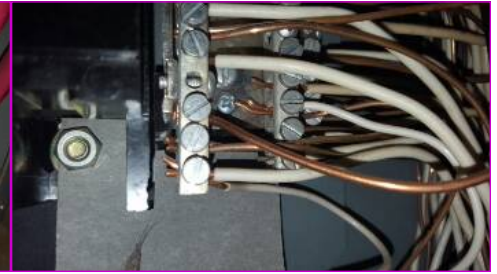
Grounds and neutrals should not be landed under the same screw in a main panel.
