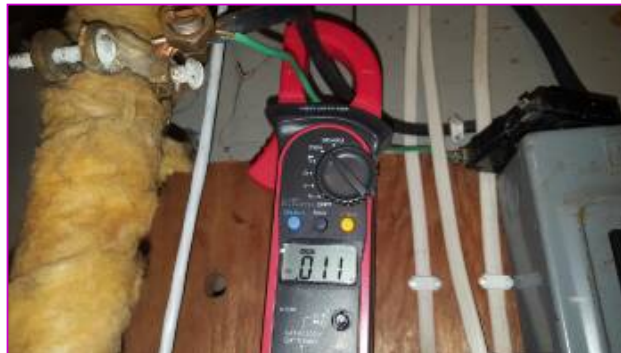
There was a small amount of current on the ground wire. Review recommended.
