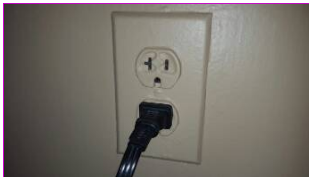
Outlets that are painted should be replaced.
