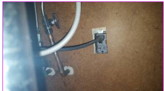
Missing cover plate.
