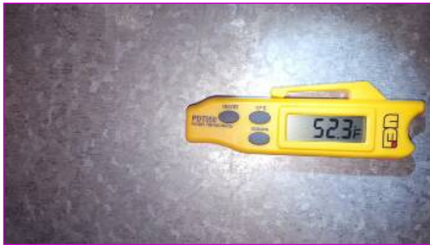
Supply air temp of 52 deg F.
