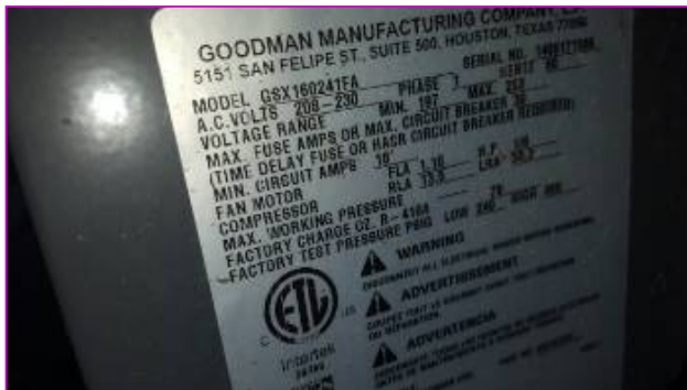
AC #2 outdoor compressor unit data plate.
