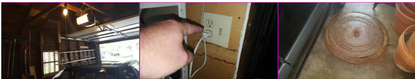
GFCI devices needed in garage.
