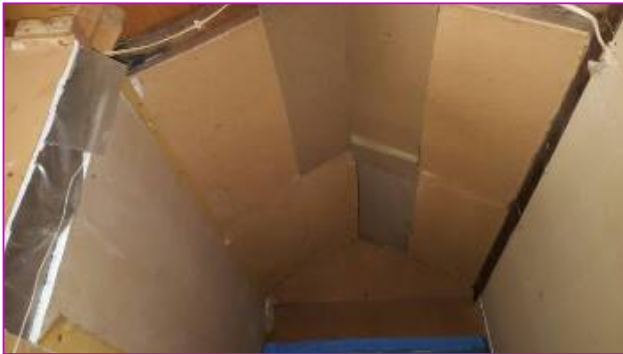
Gypsum board needed for fire separation.
