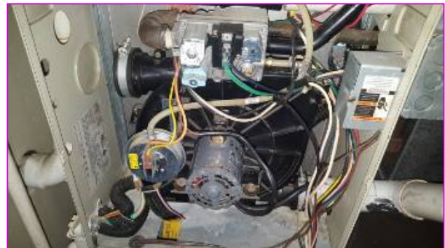
Inside furnace/ AC unit right side. Carrier Mod. 58MXA080-11112. SERIES 111 Ser. num. 2894A12909 1994
