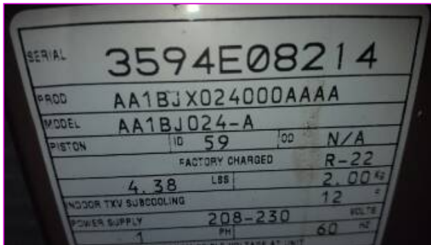
Unit #1 Outdoor compressor data plate.
