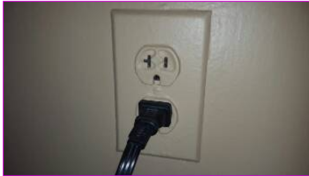
Outlets that are painted should be replaced.
