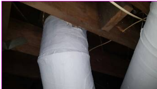
Possible asbestos duct covering
