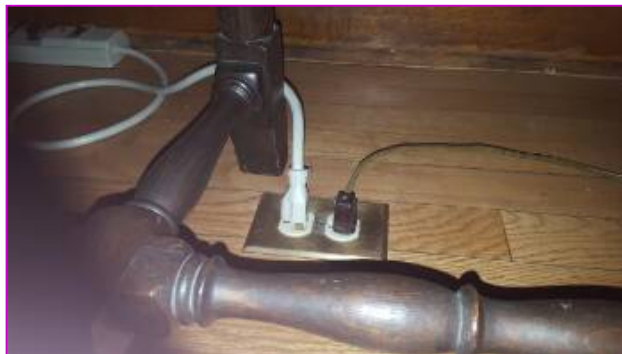
Floor outlets in the home should be replaced to protect device when not in use.
