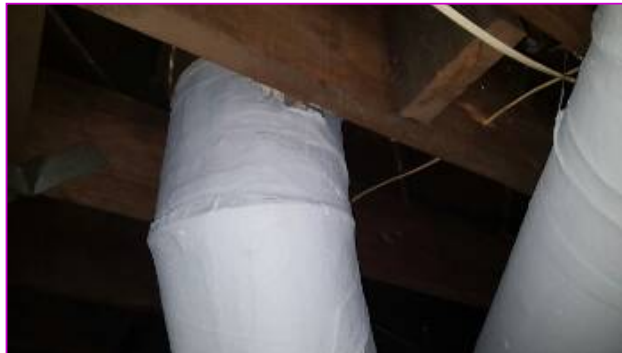
Possible asbestos duct covering
