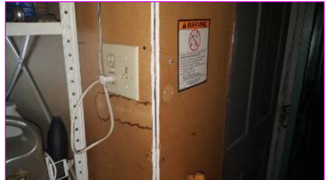
Joints should be finished for fire separation.
