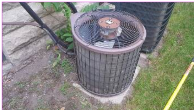
Outside unit #1 for main level of home. Made in 1994. Needs servicing.
