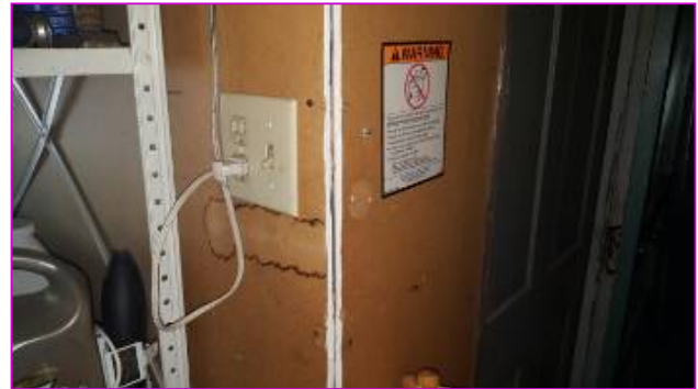
Joints should be finished for fire separation.
