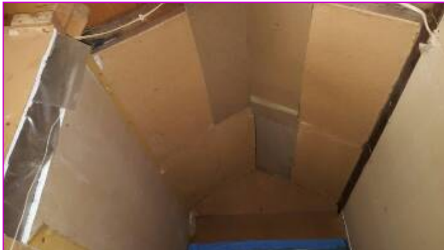
Gypsum board needed for fire separation.
