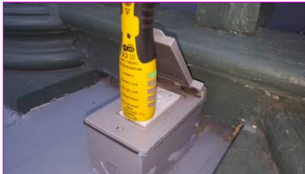
Test button failed to engage.
