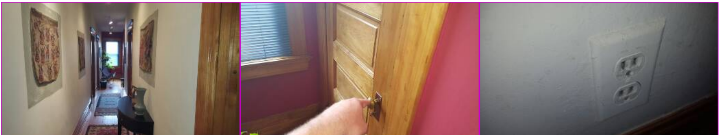
Door does not latch properly.
