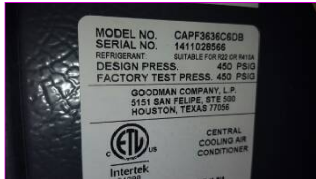
Data plate for #2 outdoor unit. Right side.
