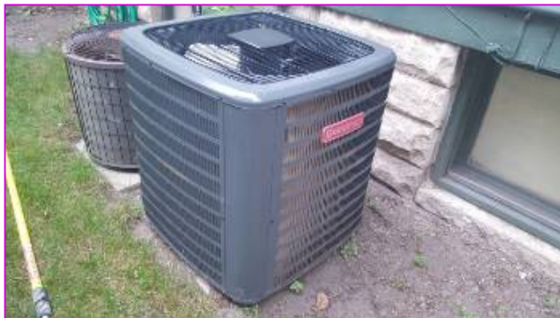
Unit #2. Services 2nd floor.
