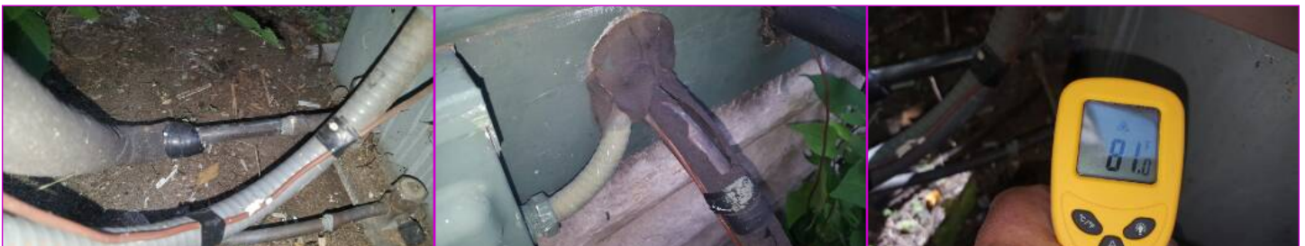
Unit #1 AC refrigerant lines.
