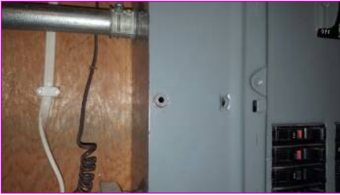
Missing panel screws should be replaced.
