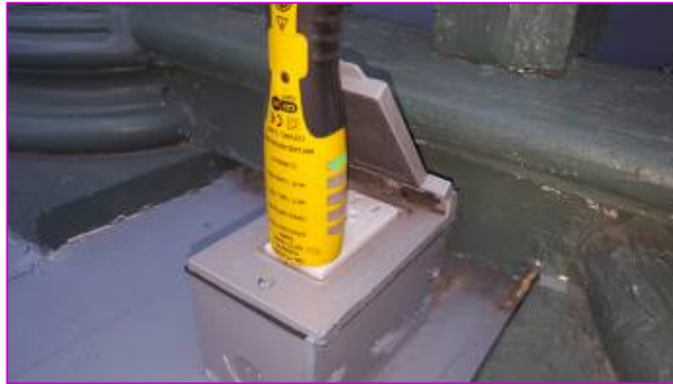
Test button failed to engage.
