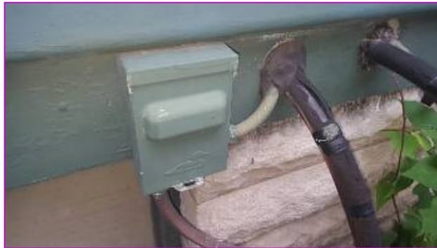
Unit #1 AC unit disconnect.
